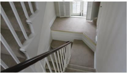
Emergency lighting and smoke detection is located in the common parts, the common part areas are showing signs of heavy wear and tear, the carpets are in poor condition and the internal common parts require redecoration. See legal section of report, you should check through your solicitor as to whether an asbestos management plan has yet to be prepared for the common parts. Such plans are mandatory with effect from May 2004.
