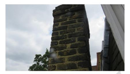
We note evidence of water ingress / high moisture meter readings internally immediately adjacent to the left hand side flank wall where the chimneys are positioned directly within the shower room area. This requires urgent investigation and repair.
