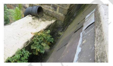
Regarding the flat roof coverings, it should be noted that compared with traditional coverings depending upon exposure, quality of felt and workmanship, flat roofs have a typical life span of 10 to 15 years. They are also prone to sudden failure and leakage. Continual maintenance and periodic re-covering will therefore be necessary. When the roofs are recovered they should be insulated and ventilated in accordance with current Building Regulations.
