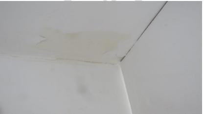
We note there is evidence of water staining to a number of the ceilings, in particular above the door within the reception room, we note the position of the boiler / plumbing installations above and this will need further investigation and repair. Water damage has affected the access hatch in the ceiling of bedroom three with similar water staining within the built in cupboard to
