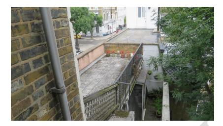
A brick parapet wall is featured to the front of the terrace and to the left hand side adjoining with the neighbouring terrace. To the rear there are metal painted railings with a timber trellis fixed to the building. We note that the brickwork to the front has suffered crack damage and we would refer to our comments under the main wall section of the report. This requires urgent repair.
