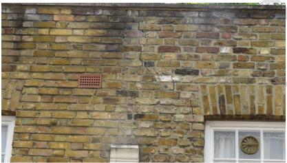
Internally there is no obvious signs of repetition of work, however these cracks will need urgent repair. We are concerned that this could give rise to damp or damage to the demise below which may also be exacerbated by the poor condition of the pedestrian covering / terrace area and it should be checked and confirmed as to whether there have been any complaints or disputes in relation to the same.
