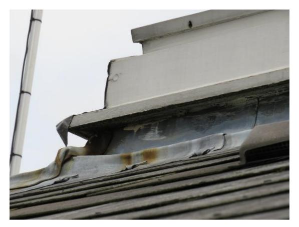
The general condition of the roof slates were found to be in serviceable condition, despite the effects of weathering. It is important to maintain the condition of these tiles, not only to secure them but to render these parts of the roof weather-tight.
