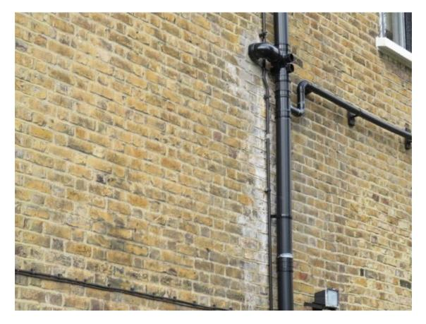
In a property of this age and type of construction there may not be sufficient restraint between the main walls and the internal elements. There is therefore the risk of bulging
