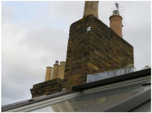
The sketch below illustrates the technology used when referring to chimney stack design. It may be seen from the sketch that a damp proof course is now incorporated within chimneys in order to prevent the downward penetration of rainwater.
